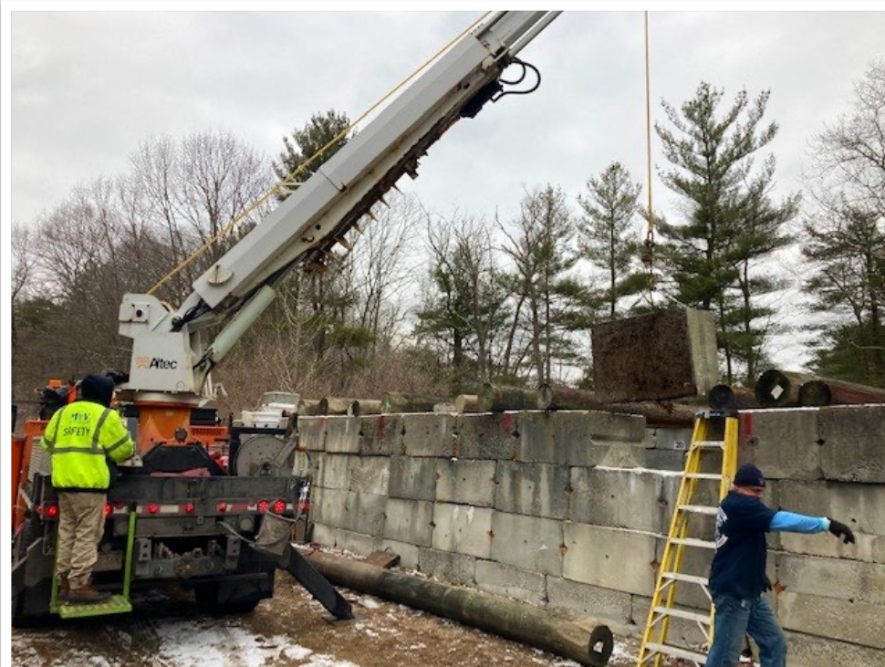
Dan Belanger removing a damaged block before the new one is installed.
